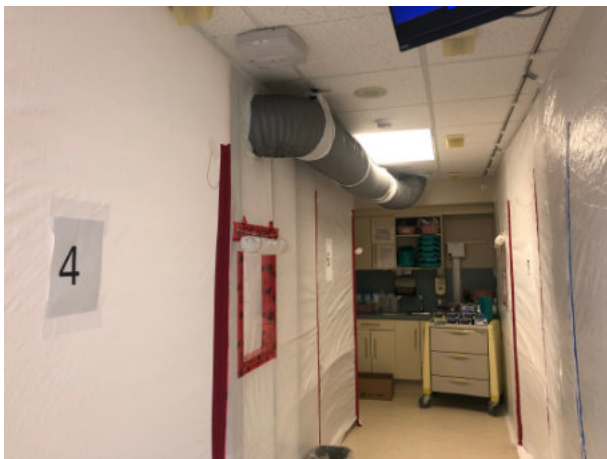
The Projects Team oversaw the conversion of spaces into negative pressure areas to isolate patients with airborne contagious diseases such as COVID-19.
