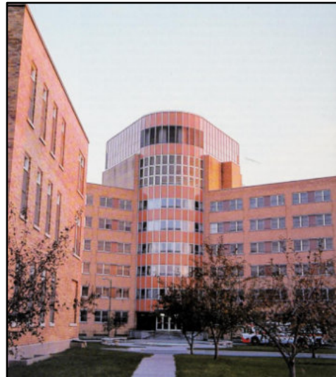
The main patient care building at Westminster Hospital in 1970, known today as Zone E 4 .
