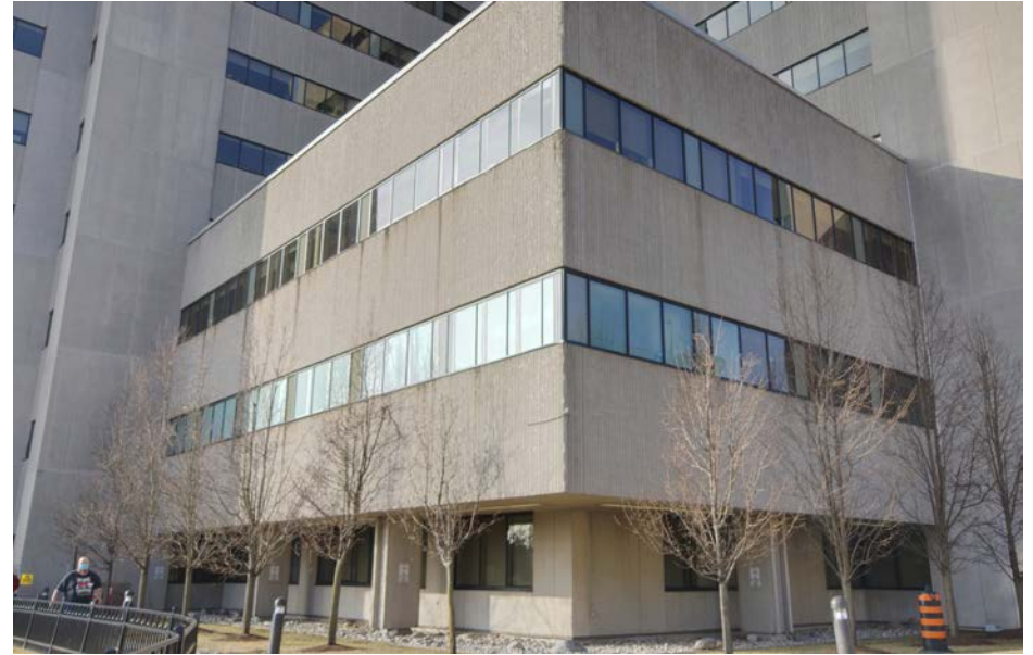
Protection against climate events at University Hospital also included new lightweight and waterproof cladding panels (below), providing protection for 24/7 operating rooms from future severe weather events.
