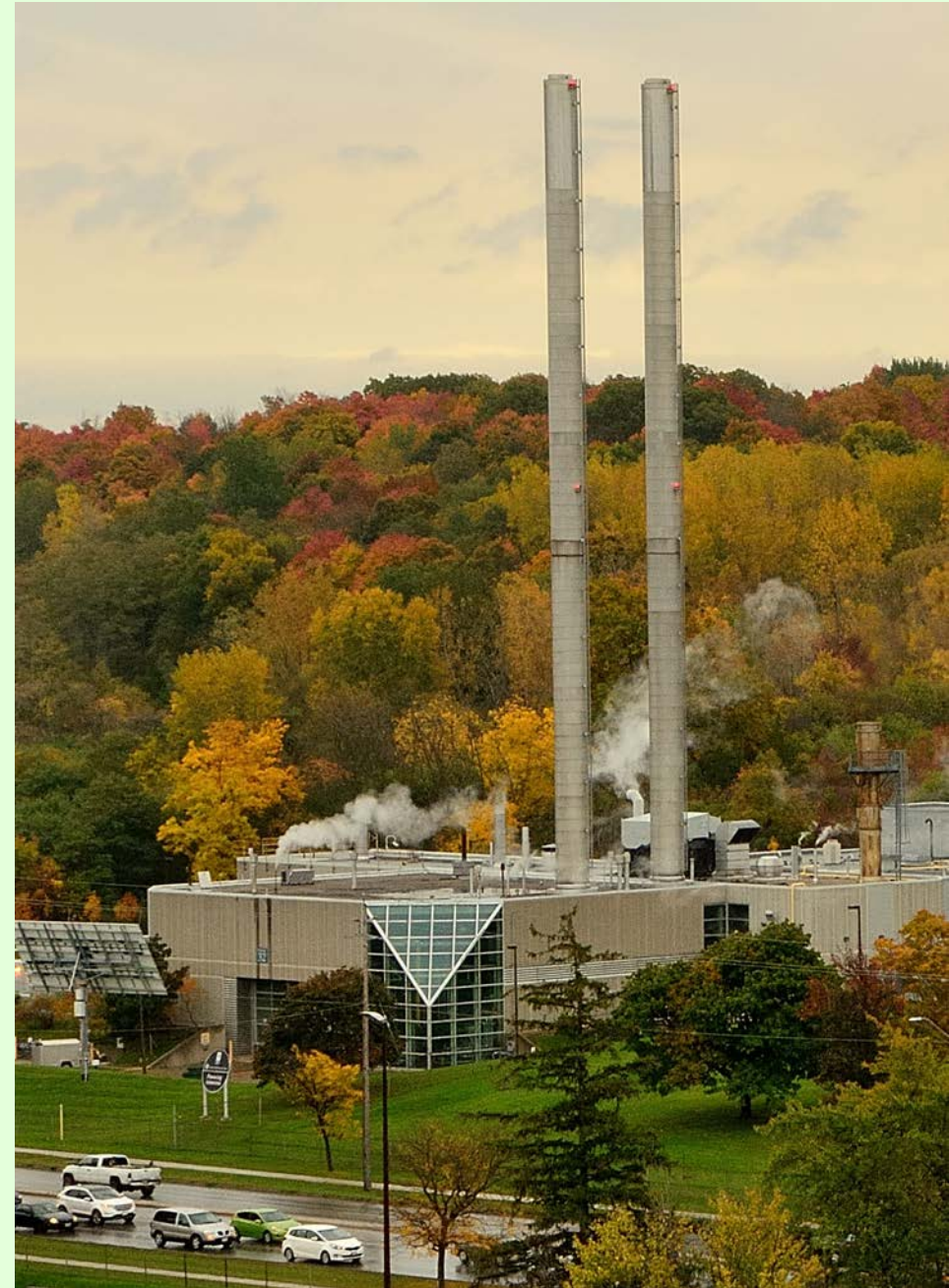
Victoria Hospital's Power Plant
