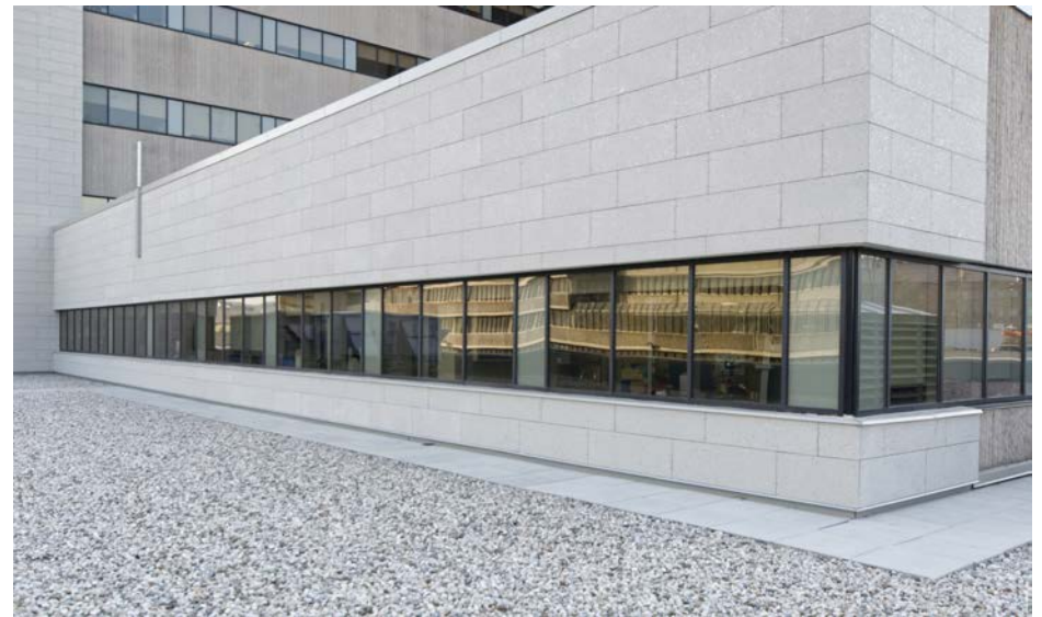
Protection against climate events at University Hospital also included new lightweight and waterproof cladding panels (below), providing protection for 24/7 operating rooms from future severe weather events.
